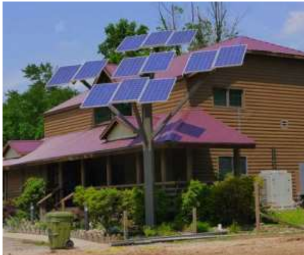
Fig 4. Mounting of Solar Tree near the house
